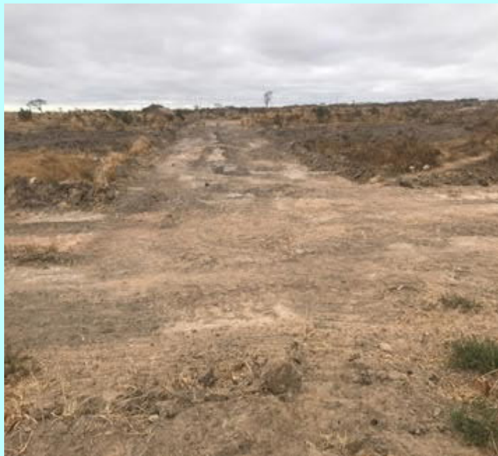
Photos showed water and road construction in progress
